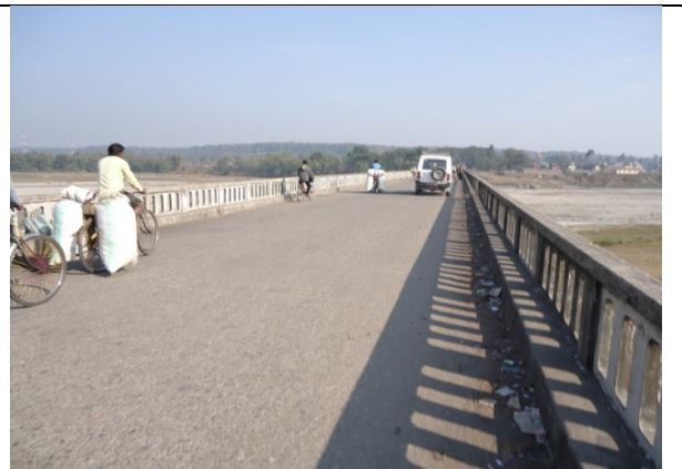
View of the Existing Bridge
